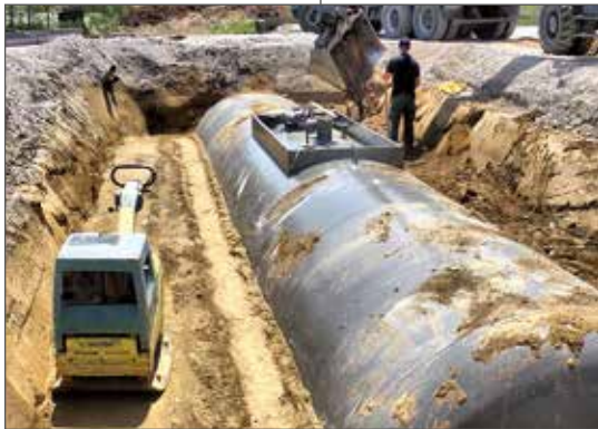
Installation of underground tank of LPG/SNG gas supply system
